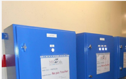
EDF - Renovation of fire detection system at 32 units
