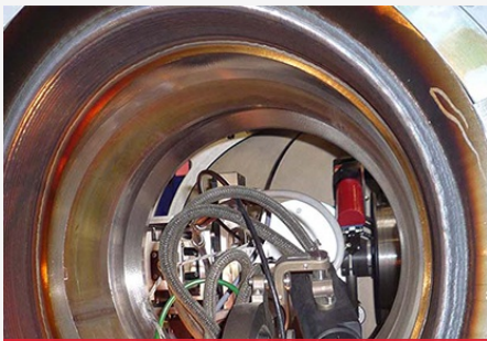
EDF-UTO - Repair of primary-side nozzles
